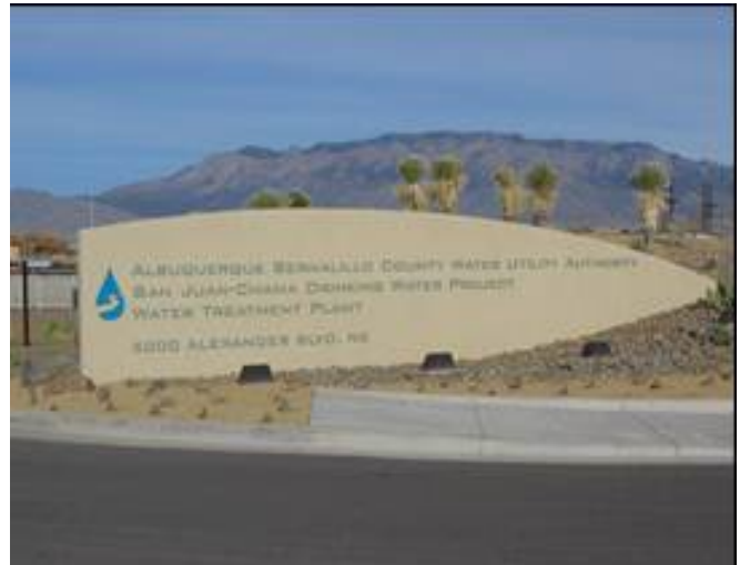
San Juan-Chama Drinking Water Plant
