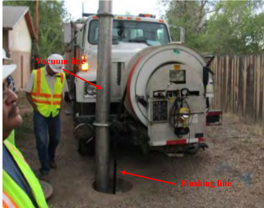
Photograph 7. Sewer System Short Interval Cleaning Crew – View of one of the Authority’s vactor trucks. In this case it was being used for short interval step cleaning.
